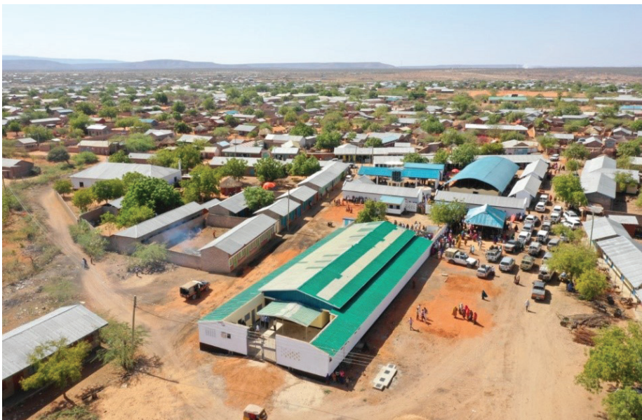
An aerial view of the Rhamu Integrated Market. October 2018 Photo | Mander County
