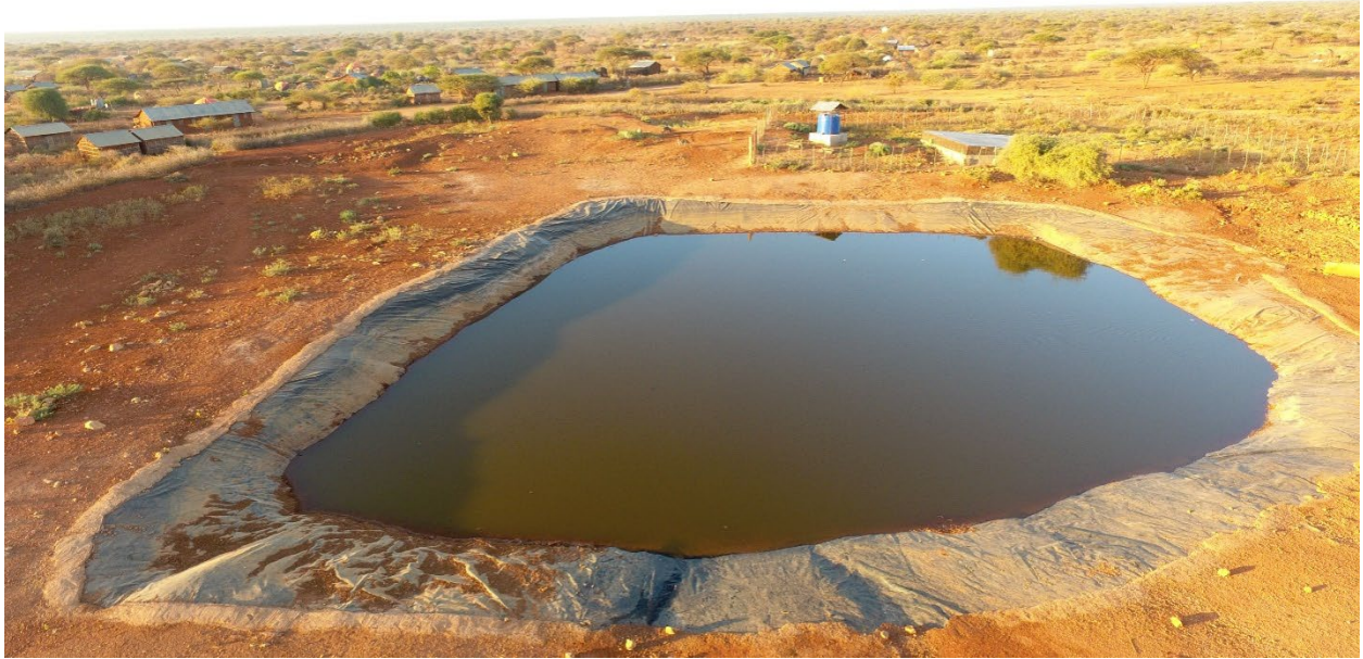
Figure 9: Malkamari water pan that was de-silted and lined in 2020 can now hold water from 4 weeks to up to six months while reducing Households walking distance by 50% in search of domestic water
